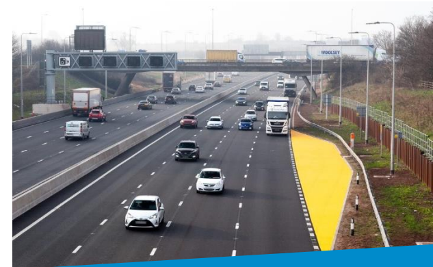
Smart motorway conversion programme
